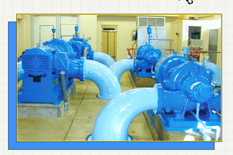
Customer was also having frequent problems with leakages due to the gland packings. This was becoming a major problem due to frequent stops, corrosion, and loss of water through gland packing.
