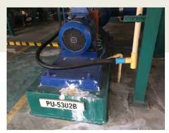
PU-5302B: Gould3196MTi Sodium Hydroxide 32%
