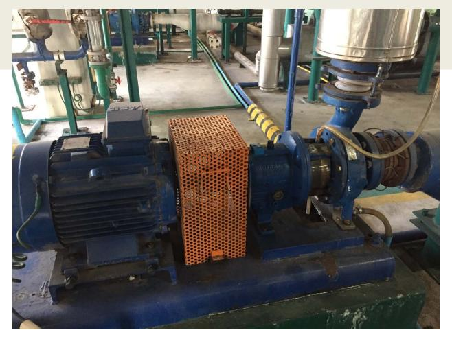
PU-5302B: Replaced to use John Crane Seal with Plan62 instead of RO Seal (Flowserve)
