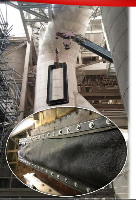
The production and service team of Townson, recently completed a major expansion joint job at a cement plant in Saraburi. The challenge was to replace 5 large fabric expansion joints within a period of 7 days. To make this possible, Townson engineers design new steel frames to make new expansion joint assembly.
