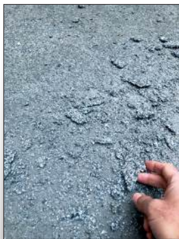
All the loose flooring material is removed
