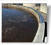
The steel plating on this clarifier tank rim, which serves as a track for the tank's scraping bridge wheels, had been in service for 15 years. Located at a Southern Louisiana wastewater treatment facility, the bridge makes approximately one full rotation every minute.
